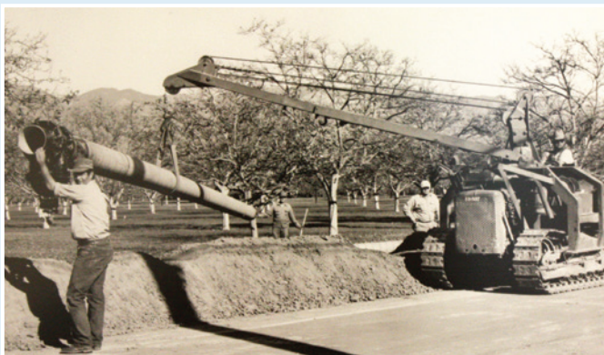
District pipeline installation in the early 1950s
