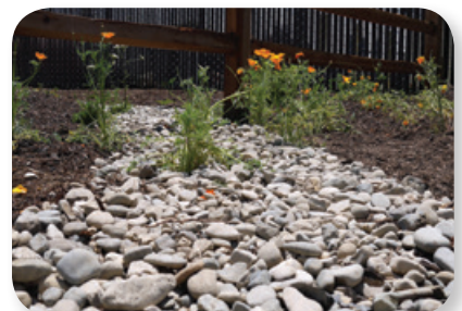
Bioswale (Dry Creek Bed)
